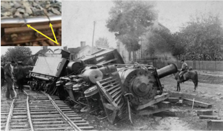
Fig. 6.9 Fracture of train wreck due to metal fatigue failure of rail from Wikipedia
